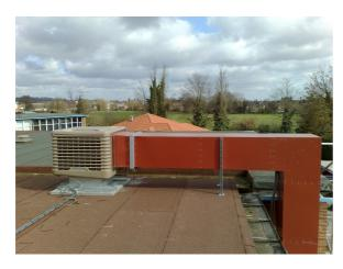
The Evaporative cooling system has running costs of less than 10% of comparable air conditioning and saves over 11 tonnes of carbon per annum.
