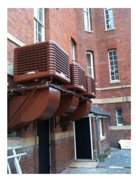
The system utilises 3 no. Celsius EcoCooling units and 3 no. wall mounted Celsius extraction units. The Celsius system has an 'atemperation' system to ensure
