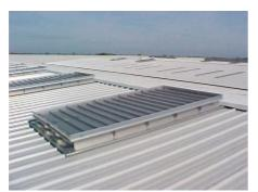
pneumatic controls, rain sensors to allow the vent to be used for a day to day ventilation and a compressor set.
