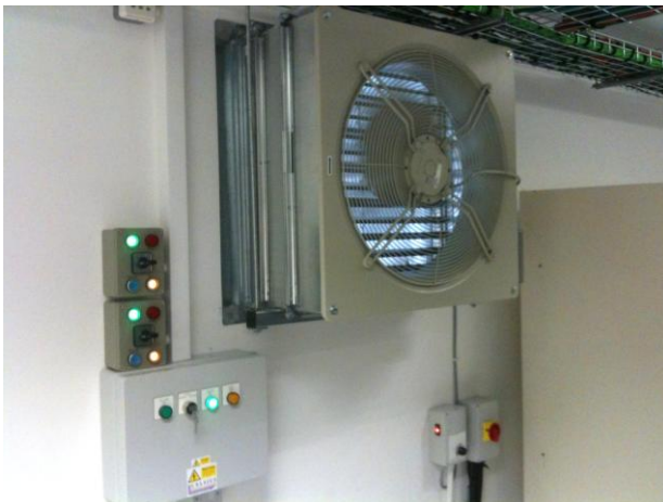
Above: Wall extraction fan and controls with dampers. Right: Detailed view of the controls.
