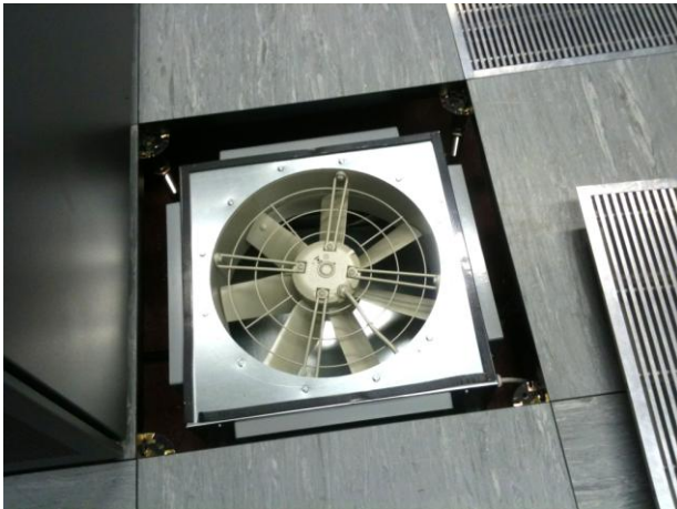
Above: Celsius underfloor atemperation fans. Right: Coolers 'squeezed' into the gap.
