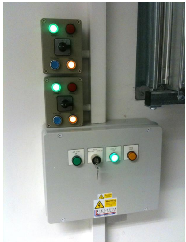
Above: Wall extraction fan and controls with dampers. Right: Detailed view of the controls.
