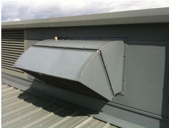
Air Intake, before the installation.
