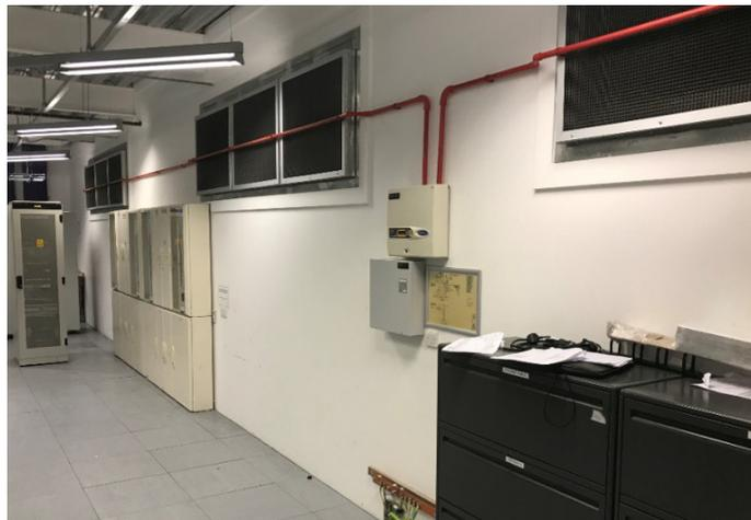
This 'alarm' is logged and reported if desired. When the smoke has passed and the VESDA system no longer detects it, the dampers alter once more to divert the airpath no longer through the HEPA filters.
