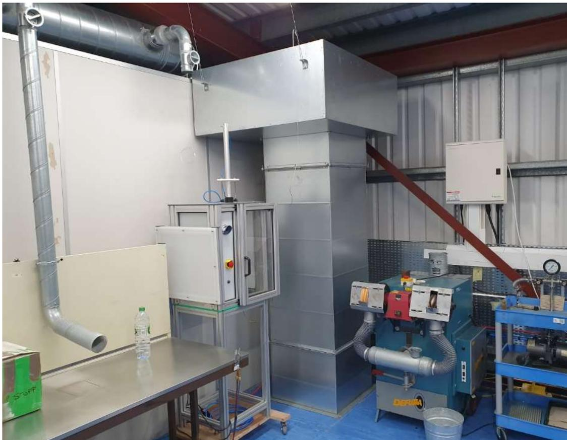
Celsius are now installing a third phase of the installation with a further EcoCooling unit on the mezzanine floor and a further Celsius extraction unit to cope with the increase in heatload from the expanded production area.
